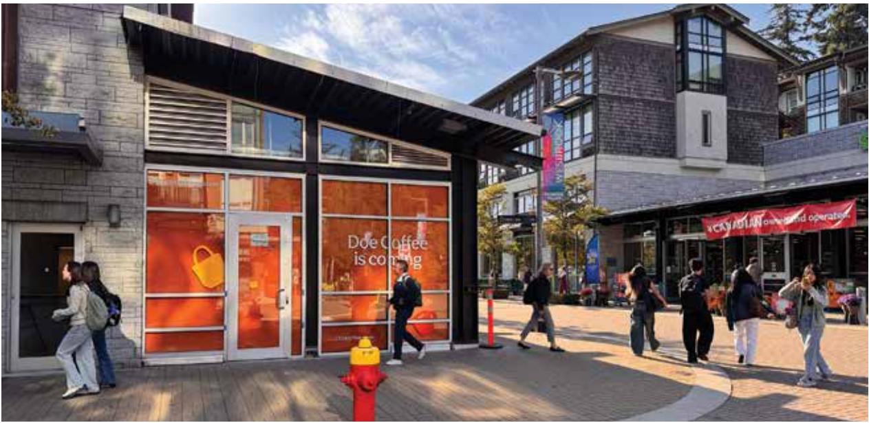
New retail space and the location of a recently-installed elevator to access the underground parkade in Wesbrook Village. (Photo: Emmanuel Samoglou)
