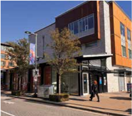
The location of the new elevator and stairway that provide access to the underground parkade in Wesbrook Village. (Photo: Emmanuel Samoglou)
