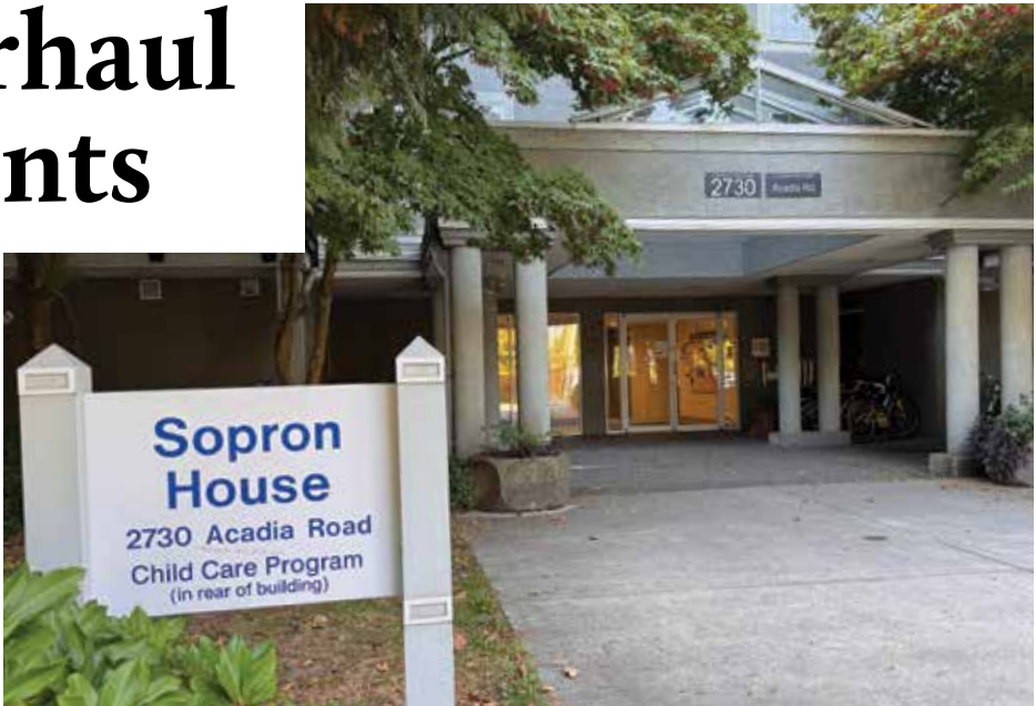
Sopron House, a residential building located at 2730 Acadia Road within Acadia Park. Residents have long complained about recurring issues with the building’s elevators. (Photo: Emmanuel Samoglou)
