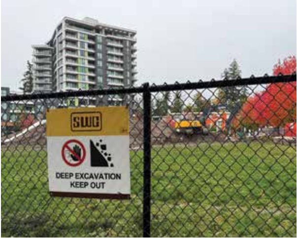
Construction underway at the southeast corner of Ross Drive and Gray Ave. in Wesbrook Place, photographed last month. Plans for the site include a 16-storey residential tower and eight townhomes. (Photo: Emmanuel Samoglou)
