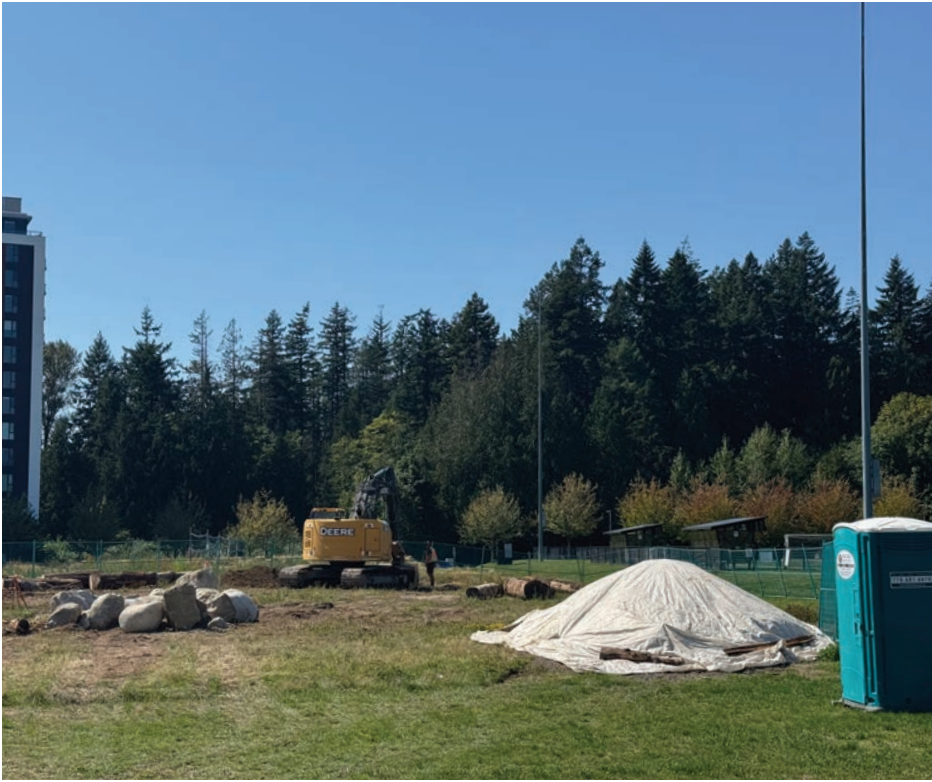
The Wesbrook Place dog park site. Construction began last month and is expected to be completed by the end of October or early November, the UNA says. (Photo: Emmanuel Samoglou)
