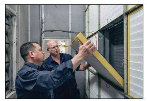
Shawn Kenney (left) and William Guest (right) from UBC Vancouver changing the MERV 13 air filters in an air handler unit located in the Pharmaceutical Sciences Building. Photo credit: UBC
