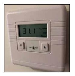
A thermostat reading of 31.1 degrees Celsius in an apartment at UBC/UNA at 9:00 p.m. during the infamous Heat Dome of June 2021. Even though the apartment had Air Conditioning, it could only cool one room. Anonymous Resident: Because balcony absorbs substantial heat from sun during day, opening windows along balcony in evening/night had minimal effect as balcony continued to radiate the heat absorbed earlier.
